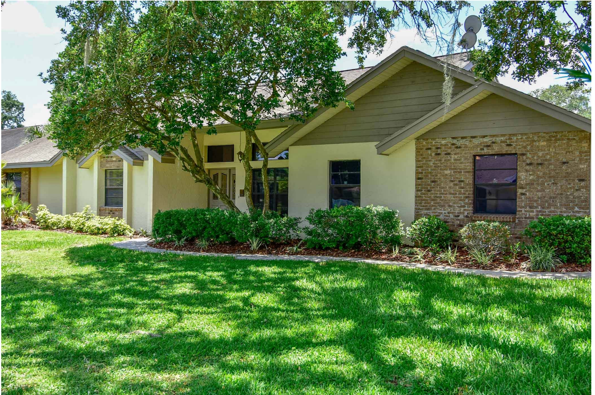
Front View – landscaped yard
