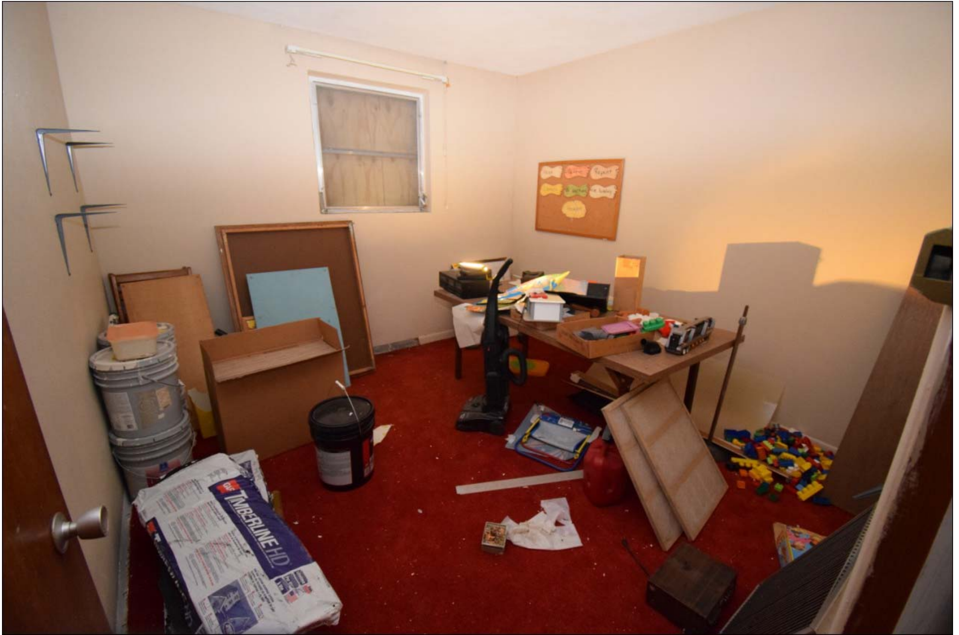
Office or Classroom 4
