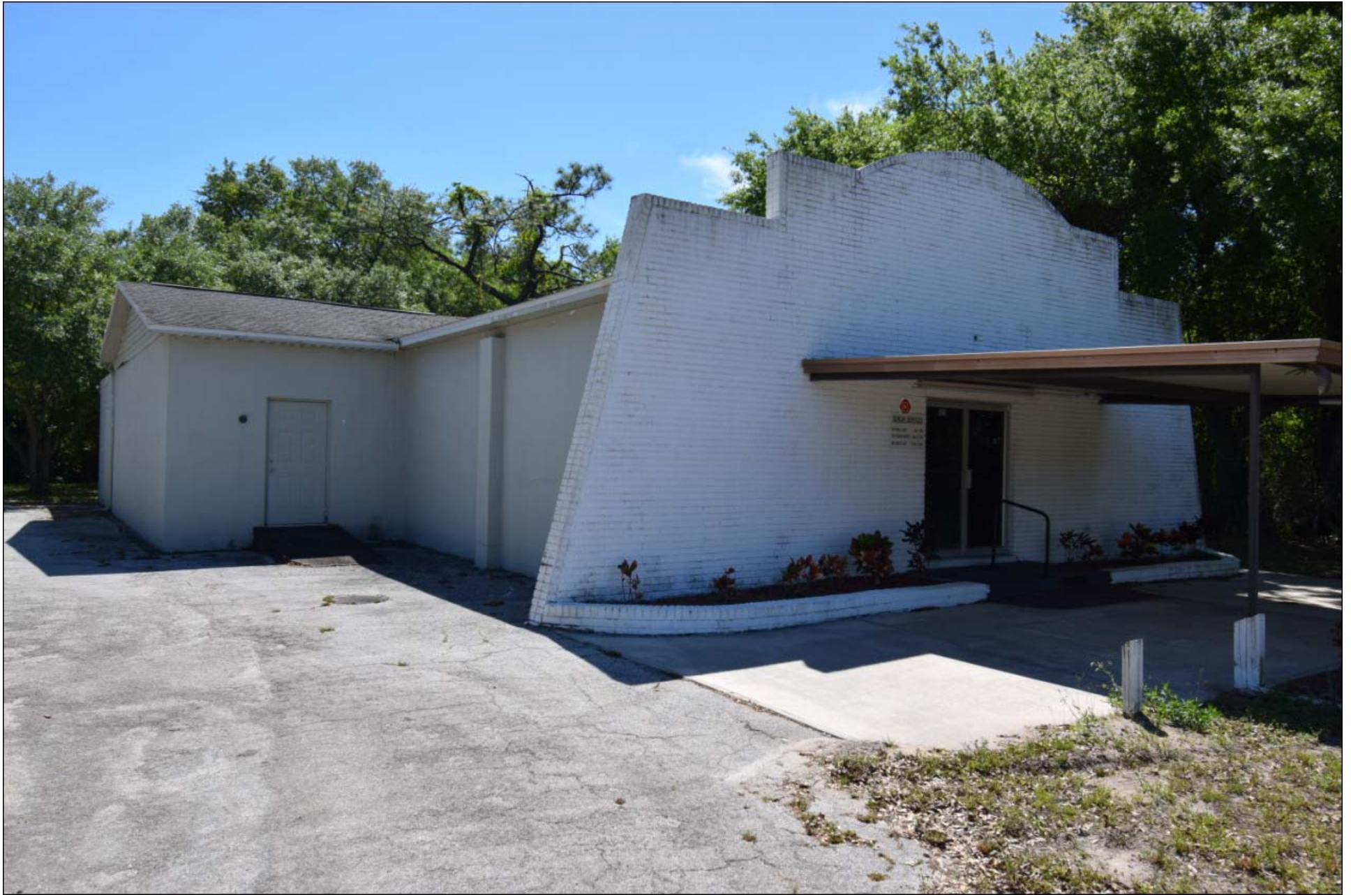
Front Entrance – Drop-off & Pick-up Canopy
