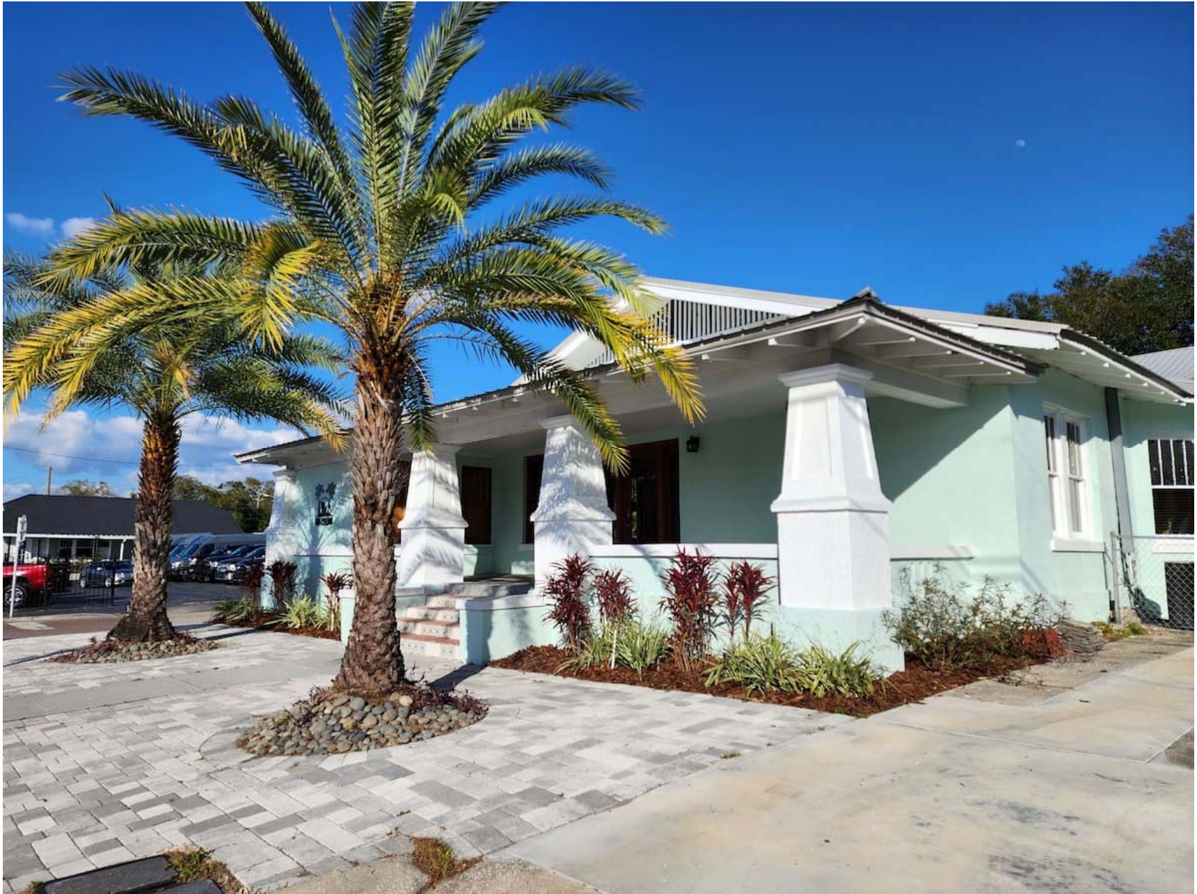
Front entrance with large porch —> 68 Pictures...
