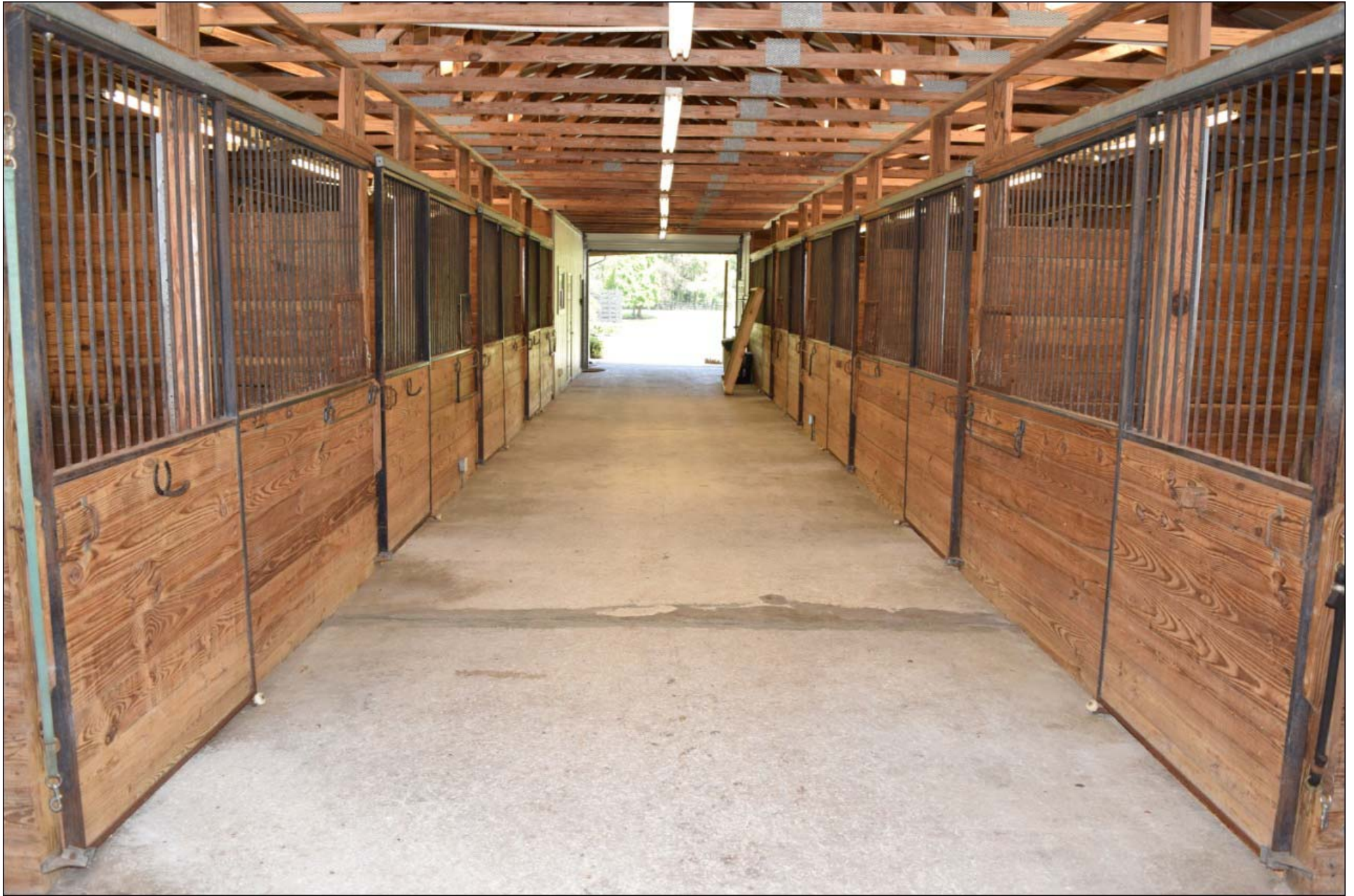
Electronic Entrance Security Gates, 21 Stalls with 'back social & cross ventilation windows' for horses calmness & comfort
