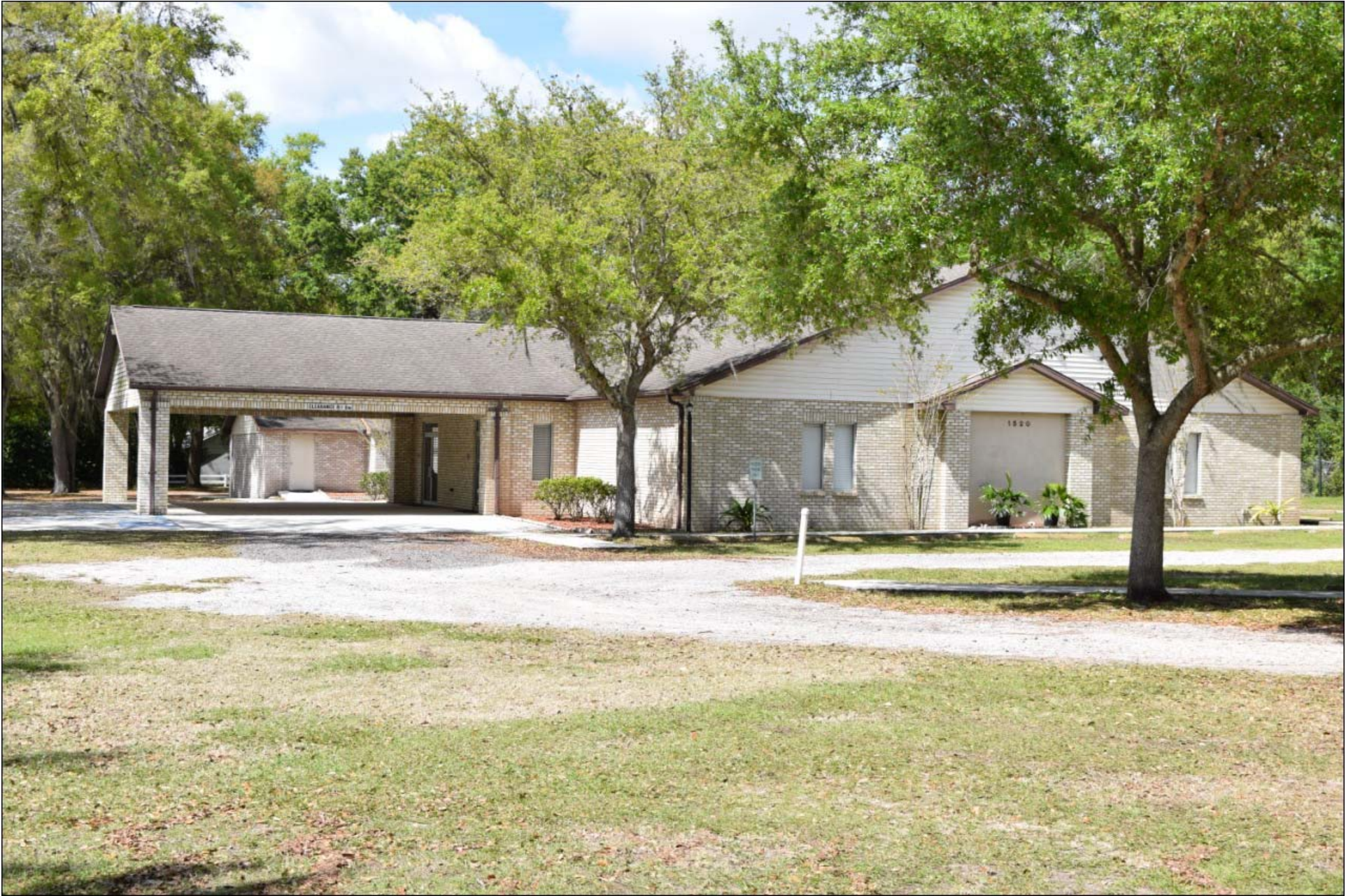
Front/Side View – a well maintained building in good condition
