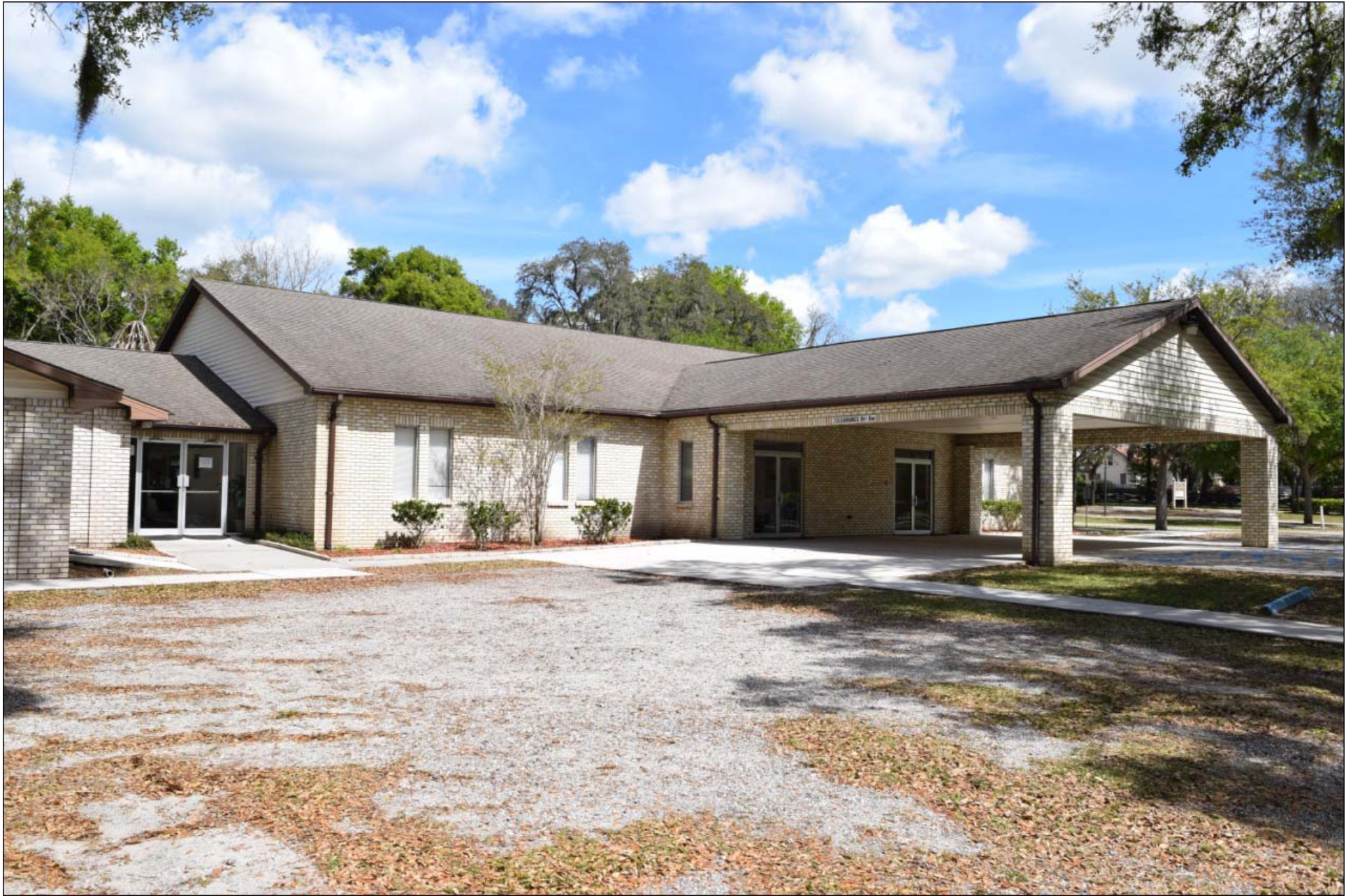
2 nd Entrance Foyer left of Main Entrance foyer
