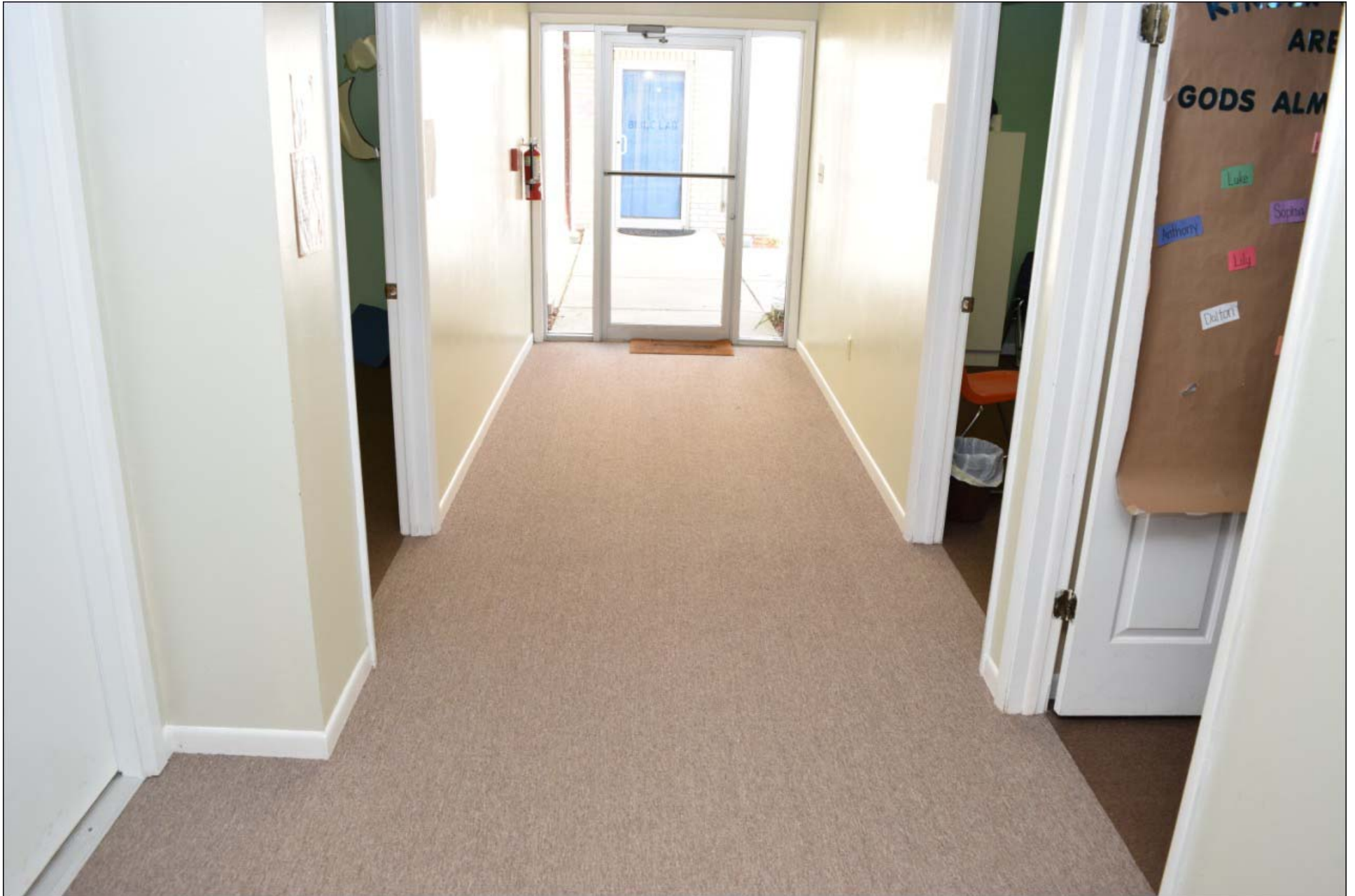
Foyer #3 with exit to building #2
