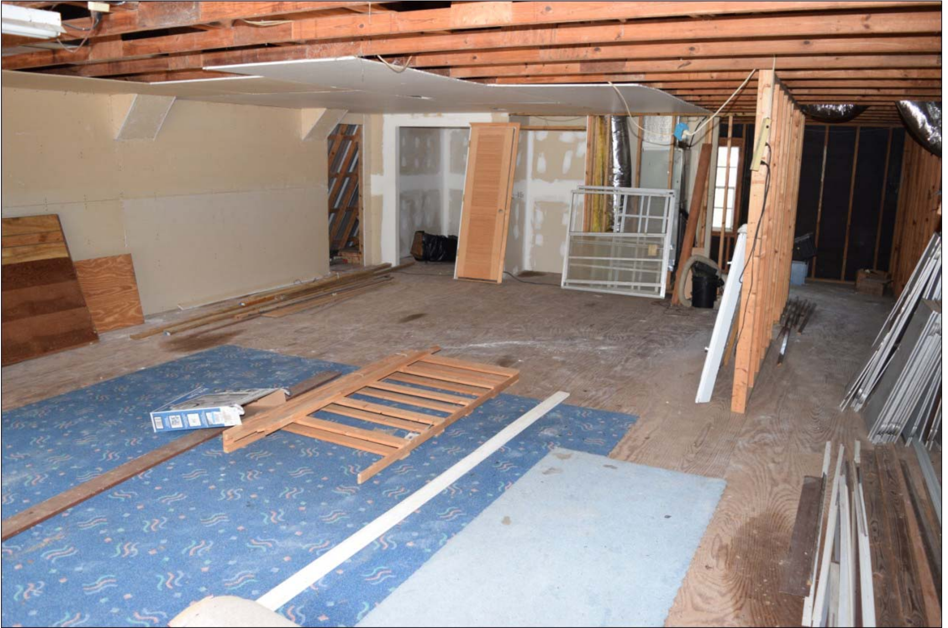
To-be-finished upstairs - under A/C
