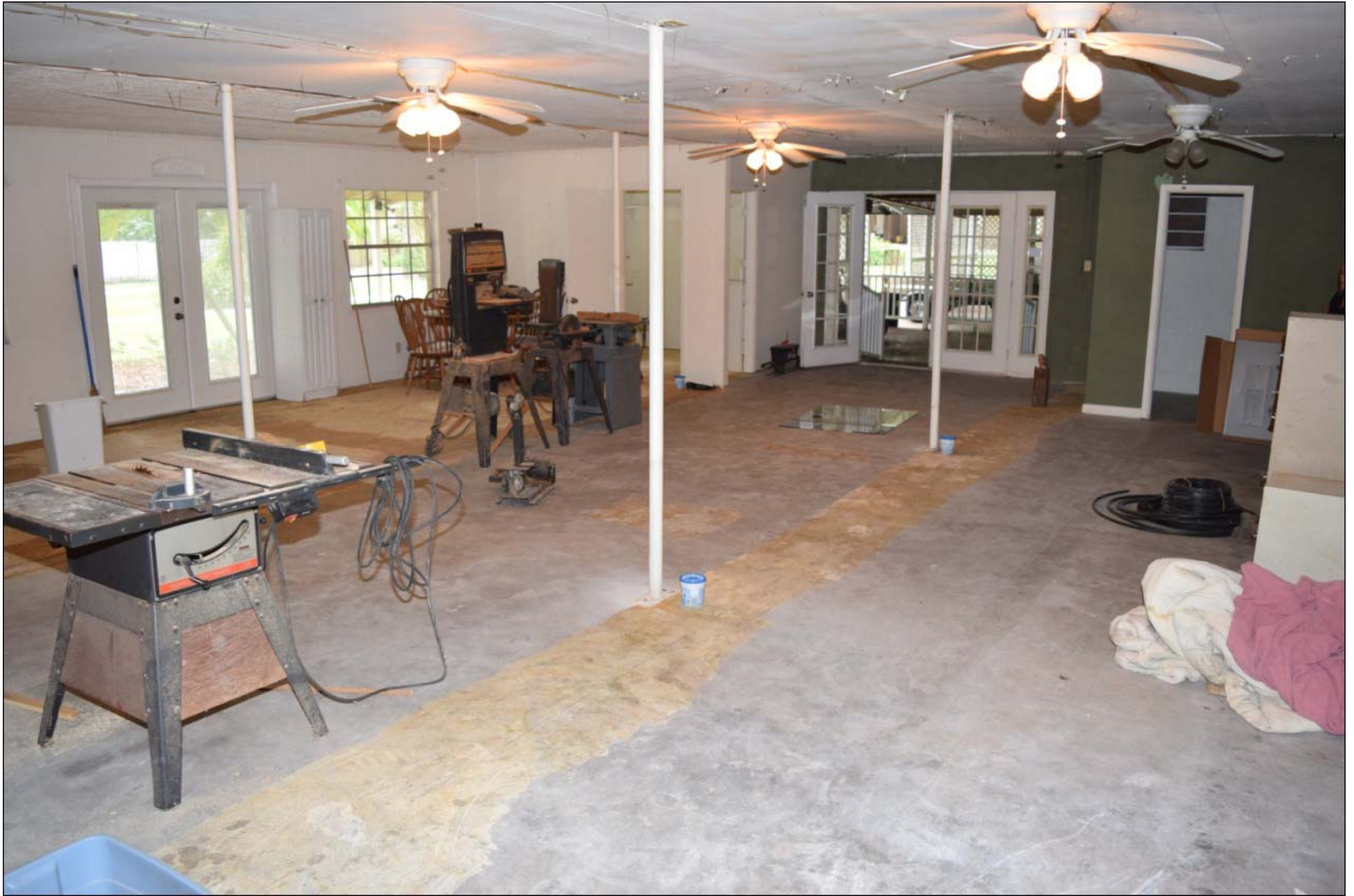
House 2 - to-be-finished downstairs under A/C - 39x33
