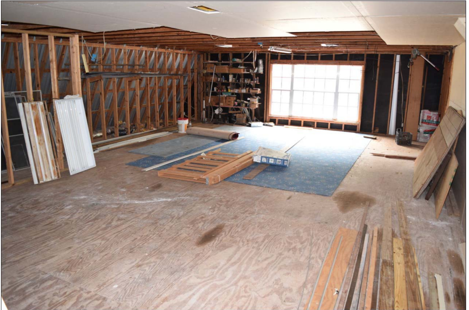
House 2 - to-be-finished upstairs with extra large window - 36x24
