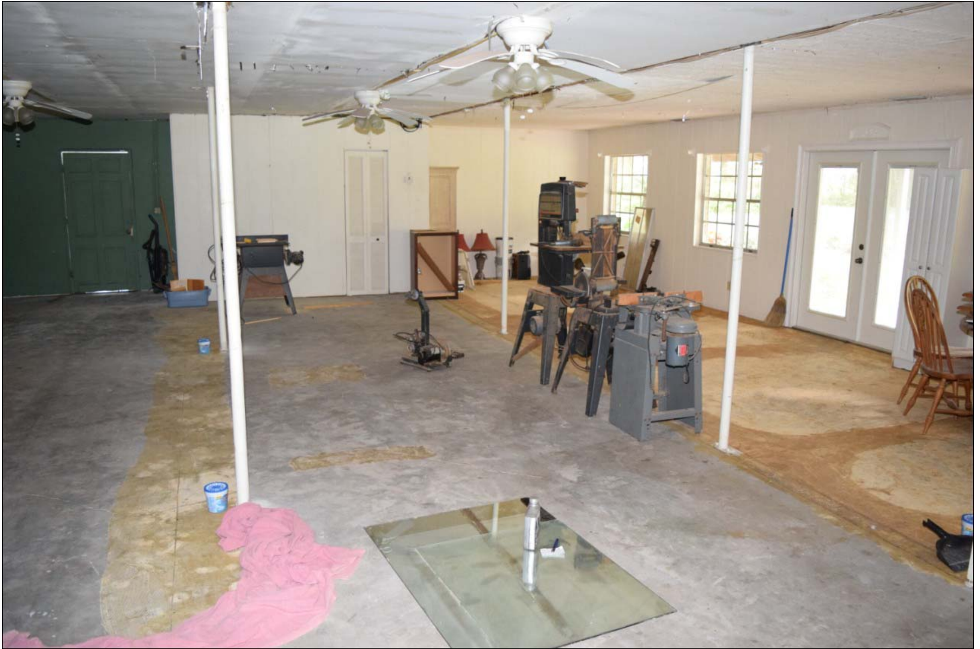
To-be-finished downstairs with Back Door & Patio French Doors
