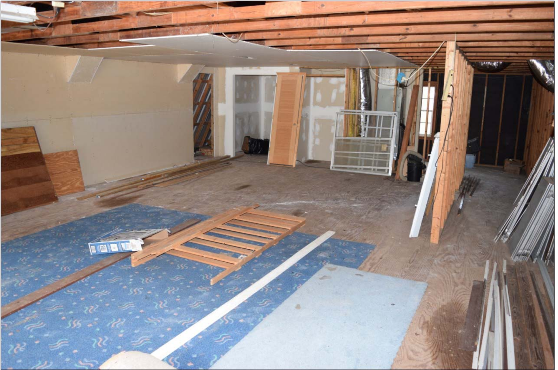
To-be-finished upstairs - under A/C
